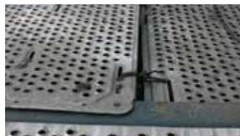
Deformed/dented and loose catwalk.
